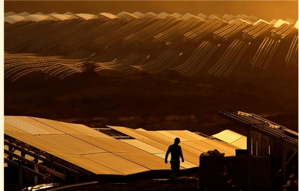
Photo: Nuñez de Balboa Photovoltaic plant - Iberdrola
